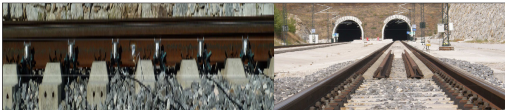
Figure 4. Geophone was installed at the study site by Crespo-Chacón et al. (2016)
